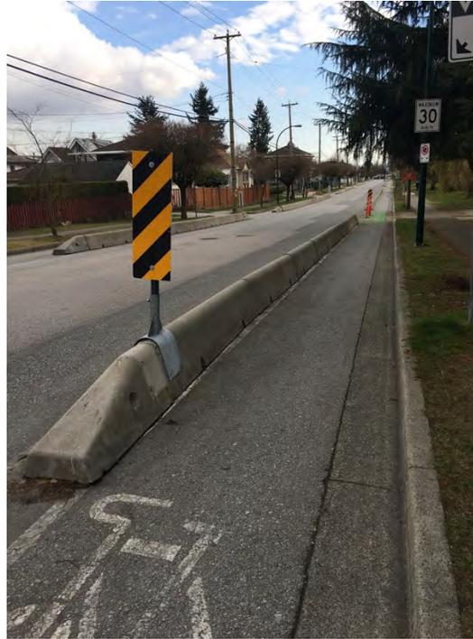
Photograph 3 & 4 - Ontario Street between 49th Avenue and 50th Avenue. This photograph shows the cement barrier that is used to protect the bike lane. While the cement barrier was found to provide a sense of safety and protection from cars for the cyclists on this route, it also leads to low levels of comfort when cyclists had to pass or be pass by other cyclists using the bike lane.
