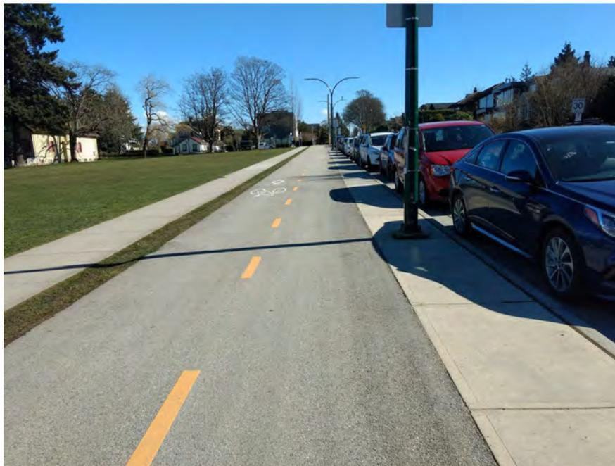
The bike lane is smooth, flat, wide, and free of obstacles. There is also a distinct separation between the pedestrian sidewalk, the bike lane, and the road. The physical barriers on either sides of the bike lane, separating the bike lane from the sidewalk and the road, increase the perception of safety for cyclists.
